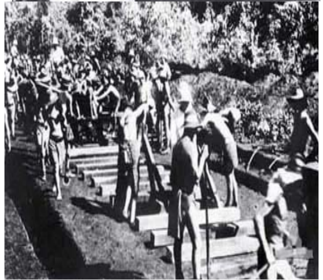
Burma Railroad. It cost a human life for every sleeper laid. 120,000 sleepers were laid.
