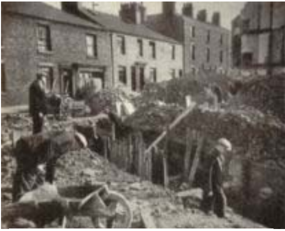
Shelters being dug in Wigan
